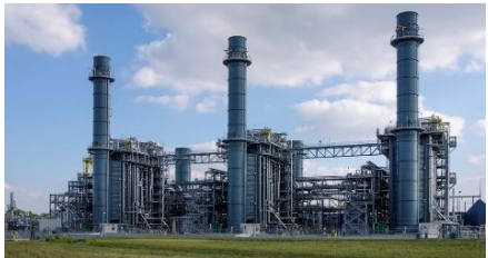
gas power plant
