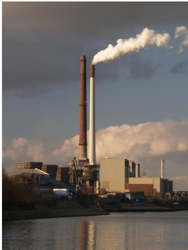
coal power plant
