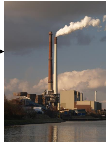
coal power plant
