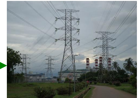
High Voltage network
